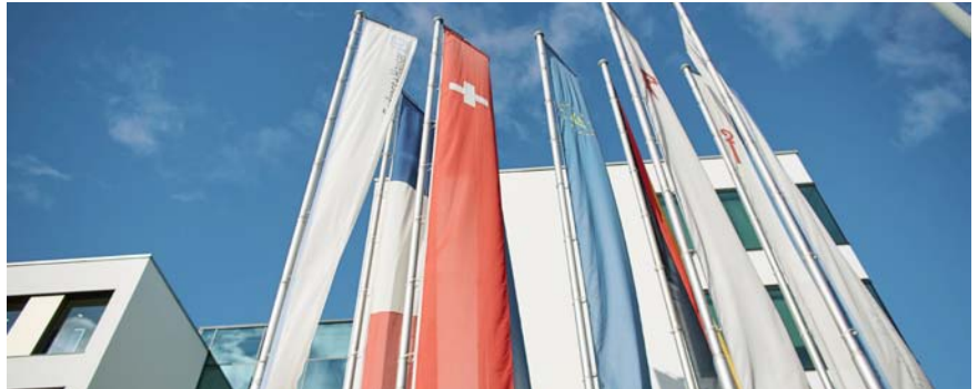
Open and transparent: The Sternenhof building in Reinach, Switzerland reflects the culture of Endress+Hauser
